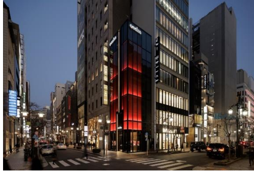
Image 1: The 5-storey Qeelin Flagship Store, situated in the esteemed Ginza district of Tokyo, exemplifies an exceptional amalgamation of architectural excellence and captivating interior design, seamlessly integrating elements of oriental cultural heritage with contemporary aesthetics.
